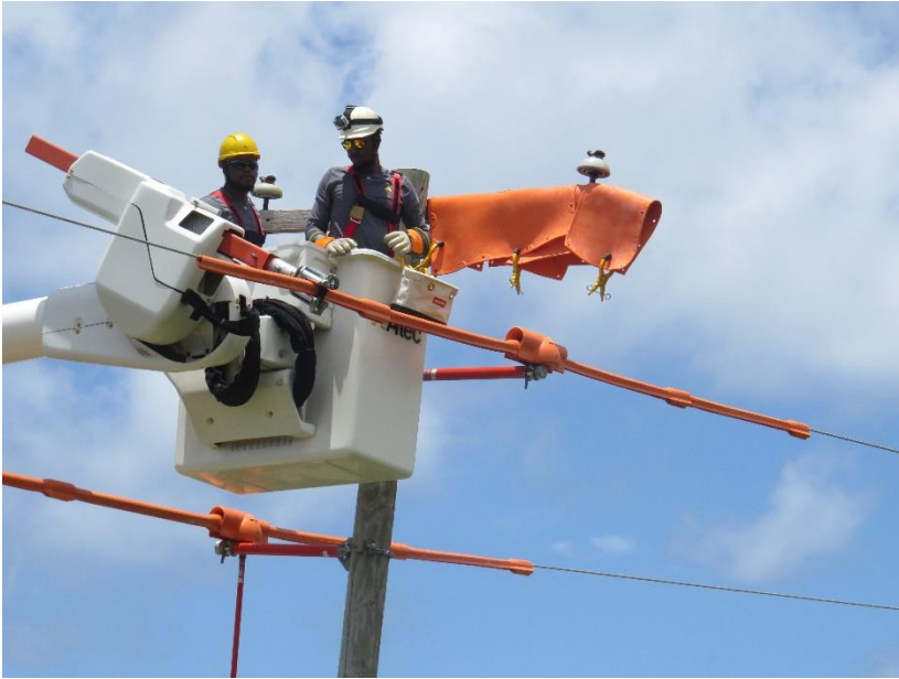
Staff performing live-line work during training.
